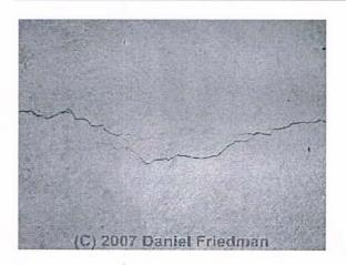
**Shrinkage cracks** in poured concrete are easily recognizable and can be distinguished from other types of cracks that occur later in the life of a foundation wall or floor slab.
